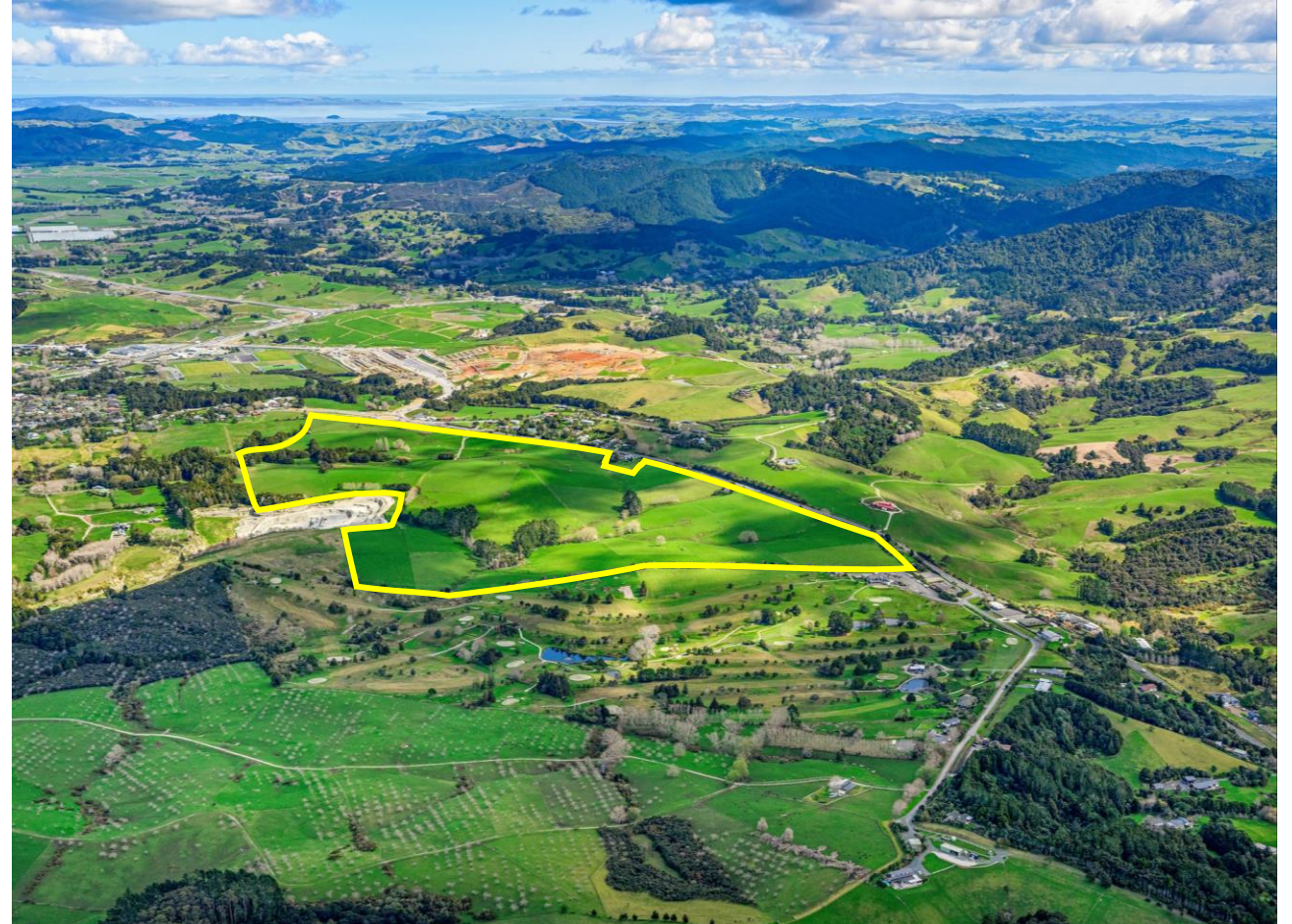
Drone image of Warkworth greenfield development site acquired in FY24. Site comprises circa 55 ha located at the end of the northern motorway, with circa 40 ha of surplus land to be sold.
